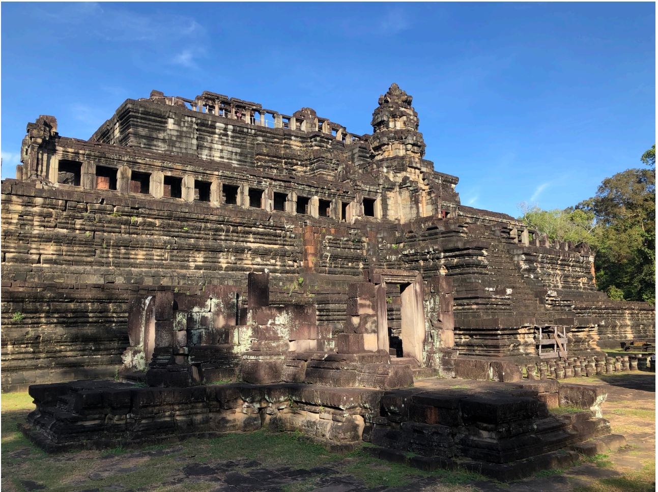
Side view of the Baphuon, from the man made hill.
