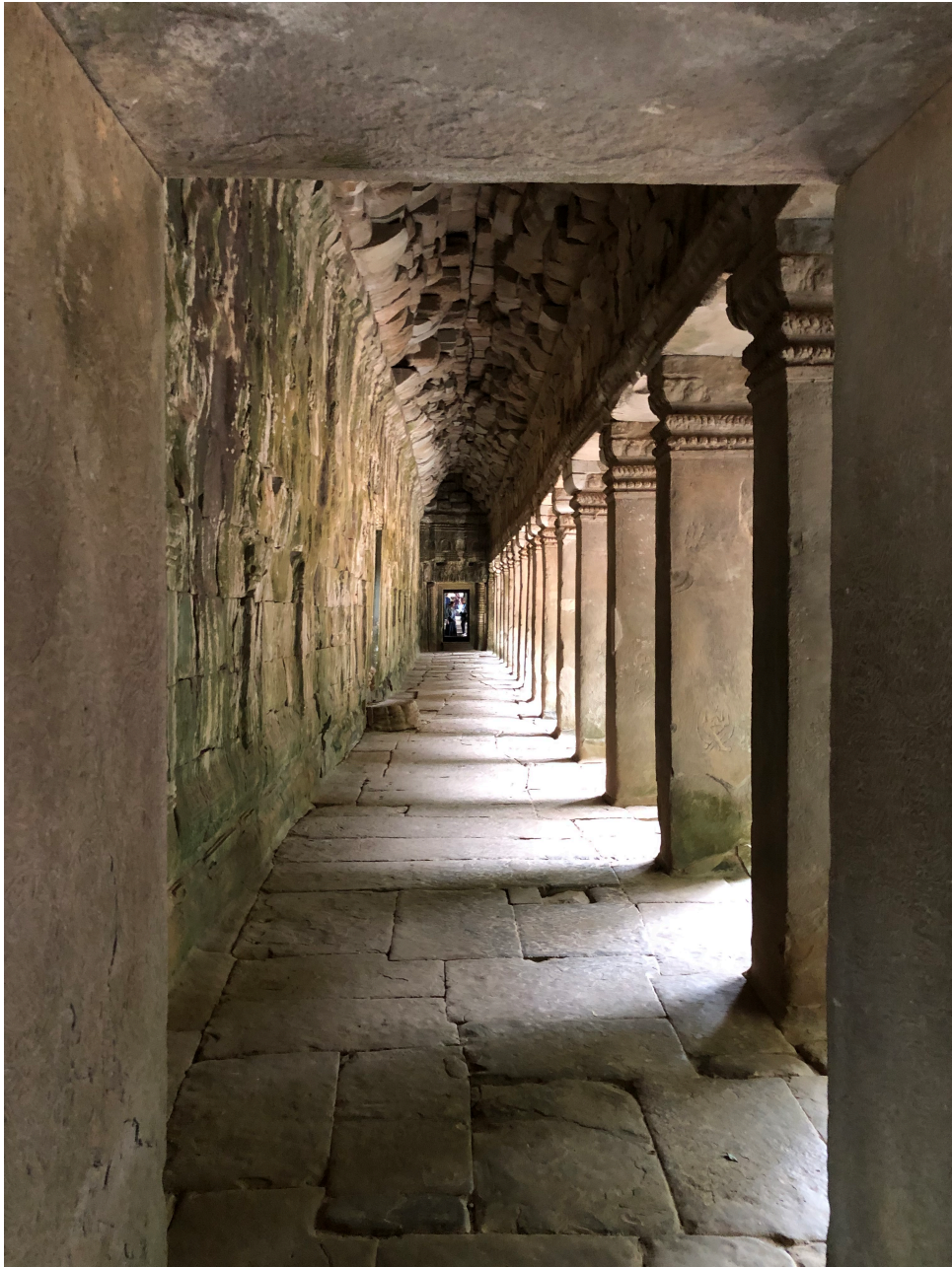
Covered walkway, east side of the temple.
