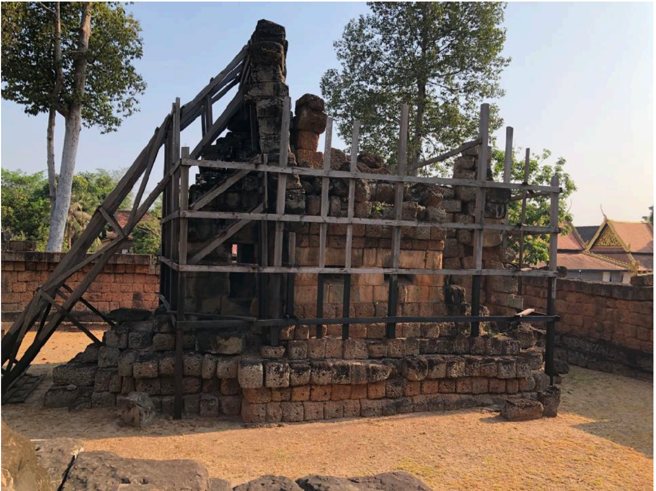
Structural support for one of the libraries and the modern pagoda buildings outside the wall.
