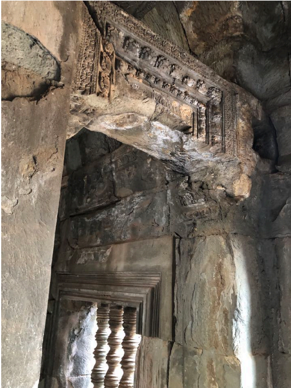
Some broken interior carvings.
