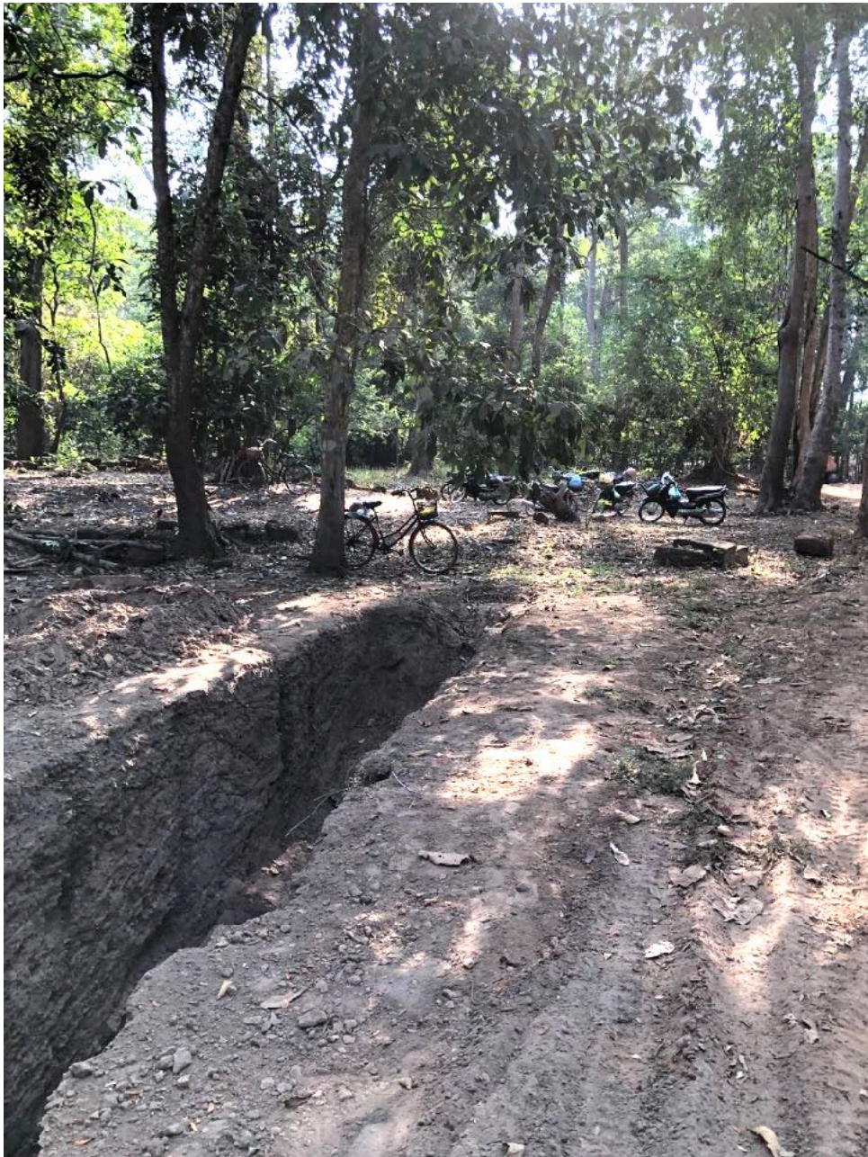
The workers' parking lot and a trench.
