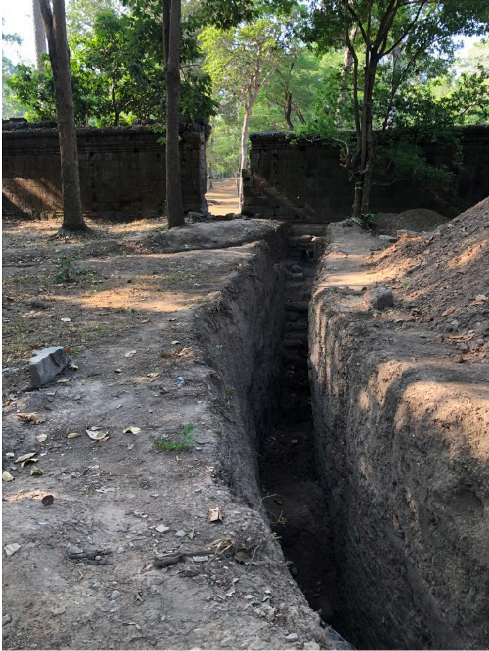
Trench and the outer wall of Phimeanakas.
