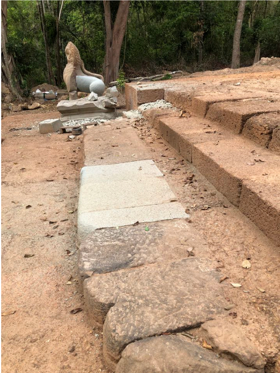
Repairs to the moonstone.
