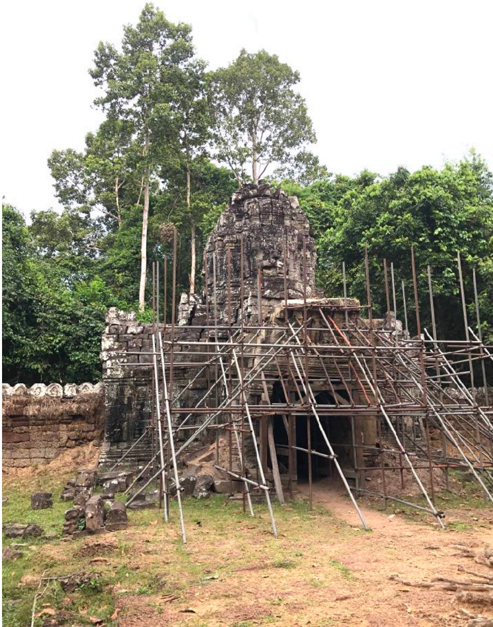
Here is the East gopura, well scaffolded, but missing the tree.
