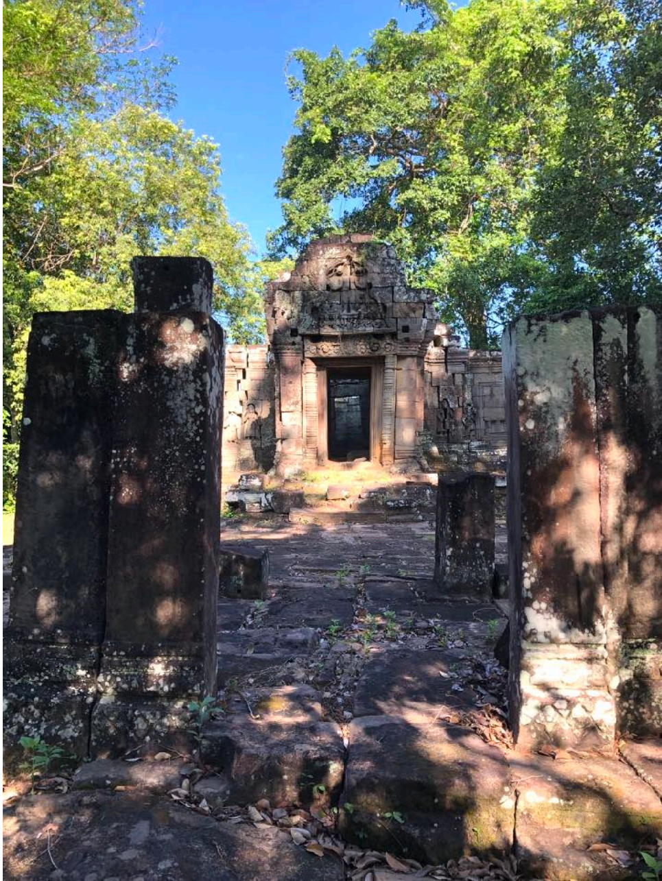
Prasat Chrung NW from the east (through the fallen gopura).
