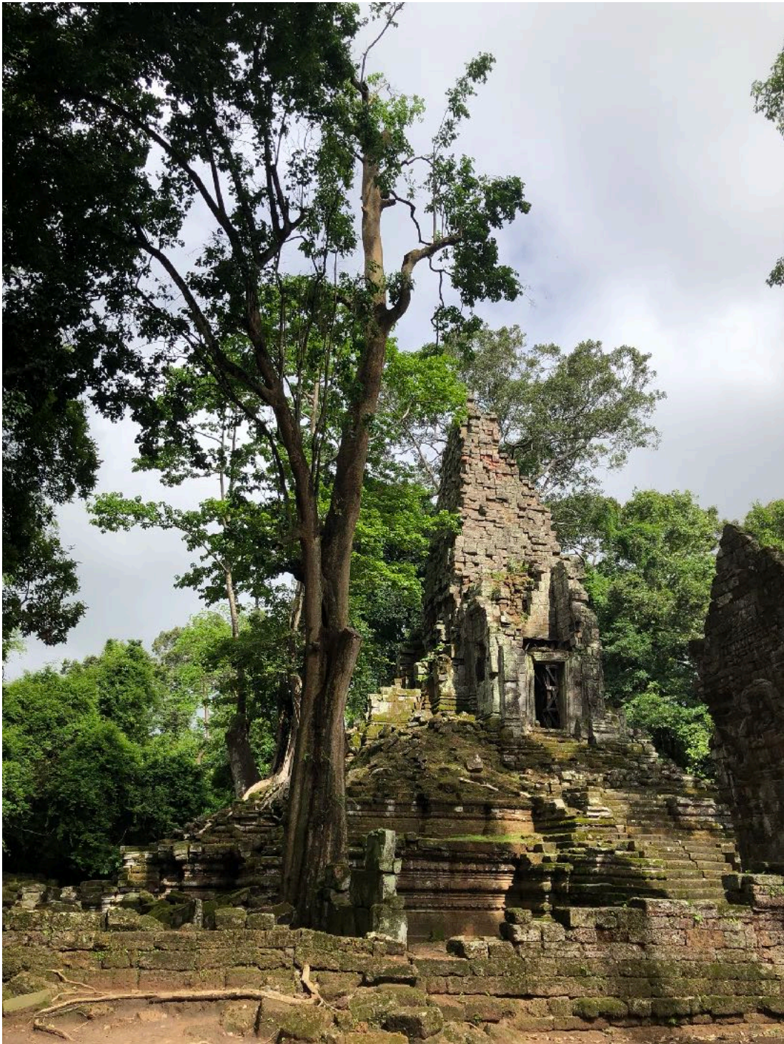
The tree near Palilay temple is now severely cut back.
