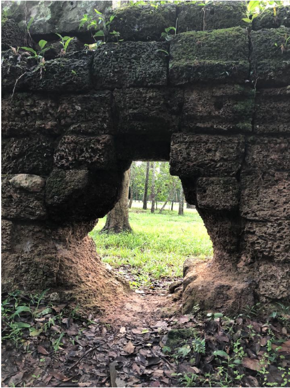
A hole in the wall, looking through to the road to Siem Reap.
